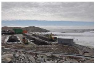
Remediation site at Casey, Antarctica showing biopile treatment cells covered in black geotextile and PRB (right)
