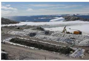
Construction of the biopile. Filling biopile with excavated contaminated soil
