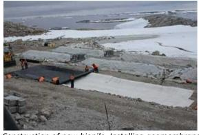
Construction of new biopile. Installing geomembrane over GCL liner
